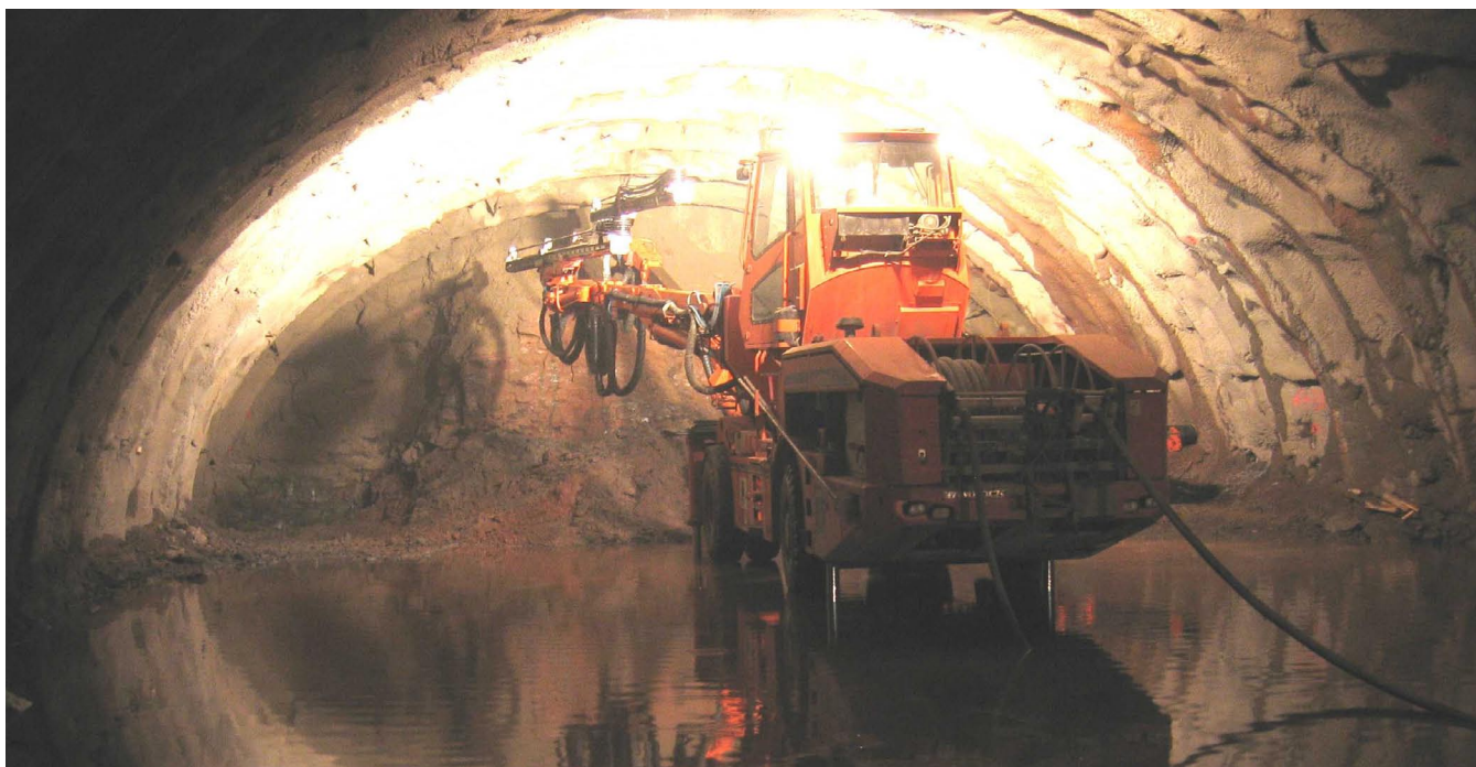
Advance drilling of Despeñaperros Tunnel with Jumbo.
